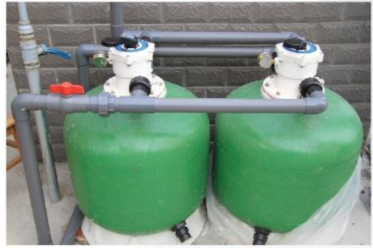
CHASSIS (Under Body) WASH SYSTEM
