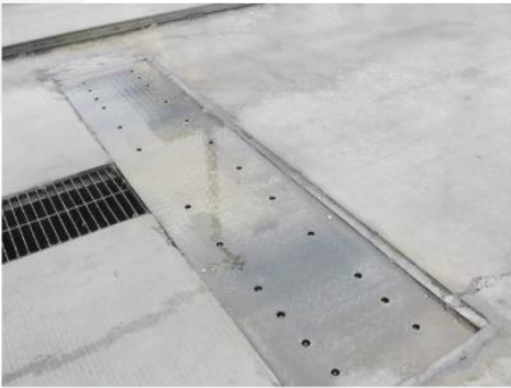
WATER RECYCLING SYSTEM
